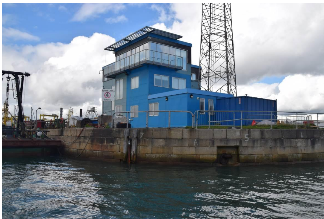
Plate 3-6 Pier Head at the terminus of Breakwater Road and the Port's Operations Building
